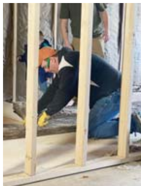
Brian Bolen cuts insulation to be installed during the construction process in 2021. The Smoldering Cigar has been open in Livermore for just over a year-and-a-half. Submitted photo.
